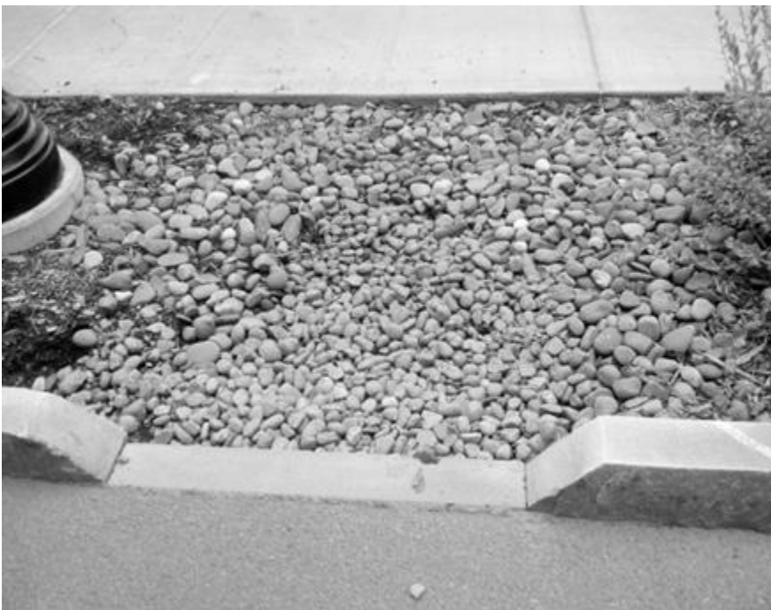
Figure 8 - Drainage at the site.
