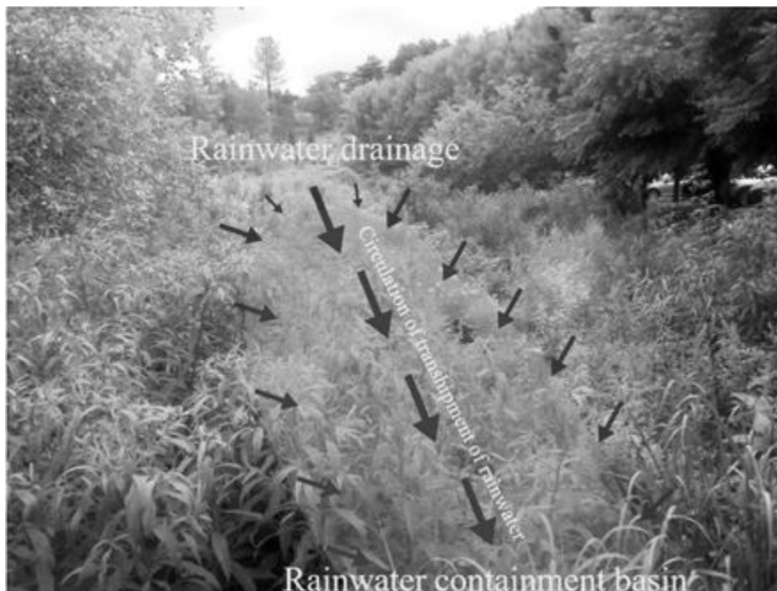
Figure 9 - Gardens integrated to the drainage system.
